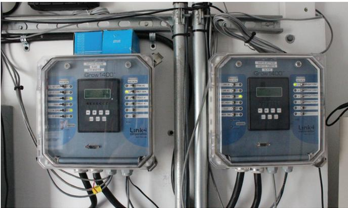
**THE iGROW CONTROL SYSTEM** is the computerized environmental control system. This is the brain of the greenhouse that allows the grower to have precise control of the heating and cooling equipment as well irrigation. The iGrow 1400 has 12 outputs and includes temperature and humidity sensors housed in special radiation housing. Also included is an outside air temperature sensor. This unit(s) is mounted and pre-wired to the electrical breaker panel.
