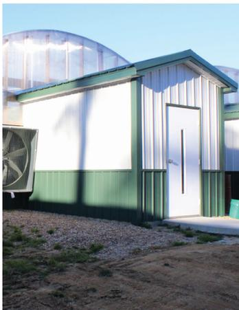
**THE HEADHOUSE** is constructed from local building materials, which adds a double entrance to the greenhouse. This is the first line of defense against pests and cold air during the winter months. A head house is a great location to place the injection system, the electrical panel, and computer.
