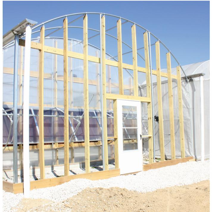
**THE SOUTH END WALL** is framed using locally purchased heat-treated 2"x4" or 2" x 6" lumber and covered in twin-wall polycarbonate that is part of the greenhouse covering package. Alternatively, the south endwall can be framed with steel purchased from CropKing, but we often find it is more economical for the grower to frame the endwalls in locally purchased, heat-treated lumber.
